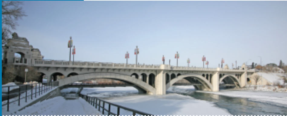
Centre Street bridge
