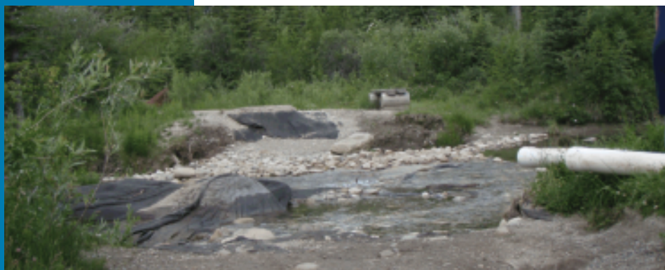
Washed out trail at Griffith Woods
